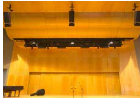
The Friends' School - curved plywood panels
