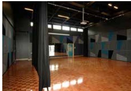
Burnie High School - acoustic wall panels
